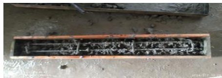
Fig. 6: Reinforcement cage
