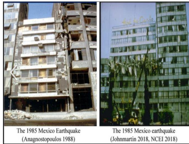
Fig .2. Effect of pounding high rise buildings
